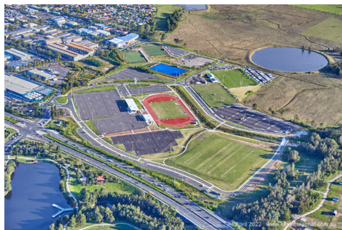
Camden Council - Narellan Sports Hub Stage 2. Image credit: TRN Group.
